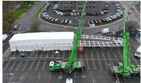
Main Span assembled in the cathedral carpark - November 2022
