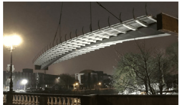
Main Span been swung into place - December 2022
