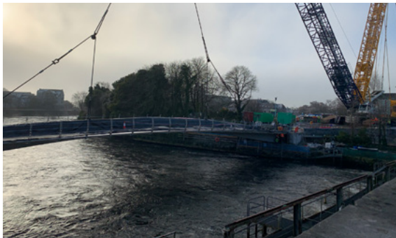
Main Span installed - December 2022
