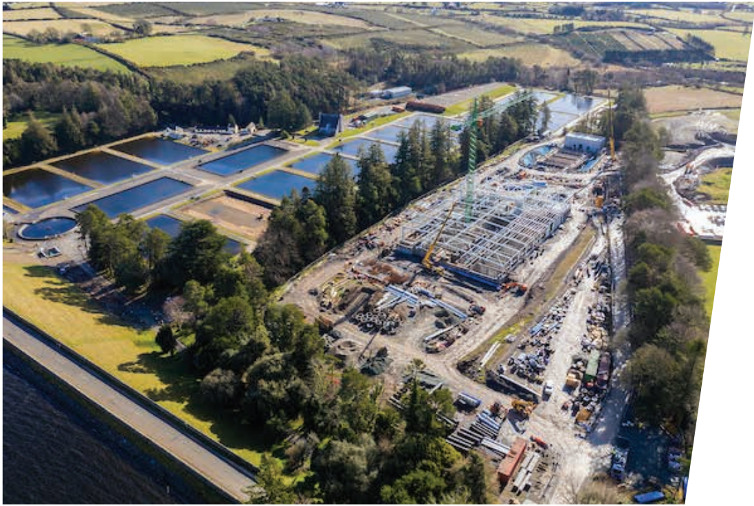
Construction of the new water treatment plant at Vartry (March 2020)
